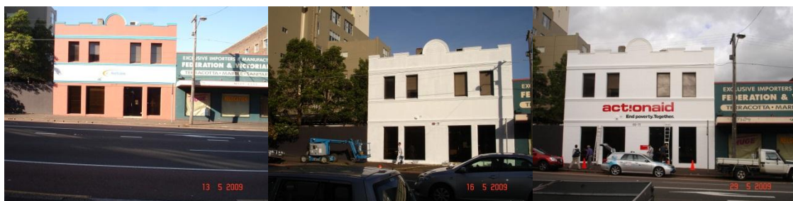
ActionAid Australia Office
